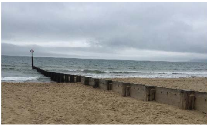
Figure 1: Timber sea defence groyne.
